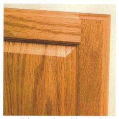
A stock frame-and-panel door. A solid red-oak frame surrounds a veneered panel. Frame pieces are joined at the corners in a cope-and-stick pattern, a standard door joint. The panel is a very thin wood veneer over particleboard, not solid wood. Some sanding marks are evident on the inside of the door.
